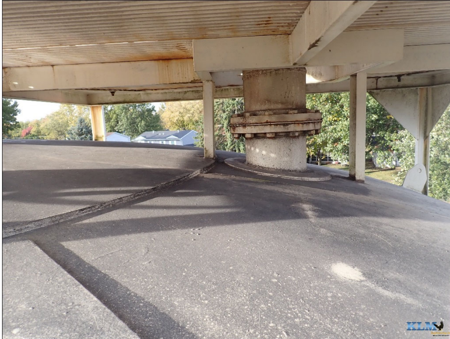
Photo No. 19 Aerator pipe and framing
