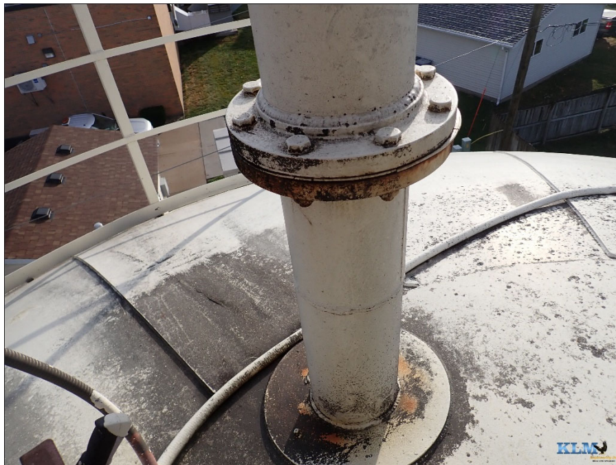
Photo No. 22 Aerator fill pipe
