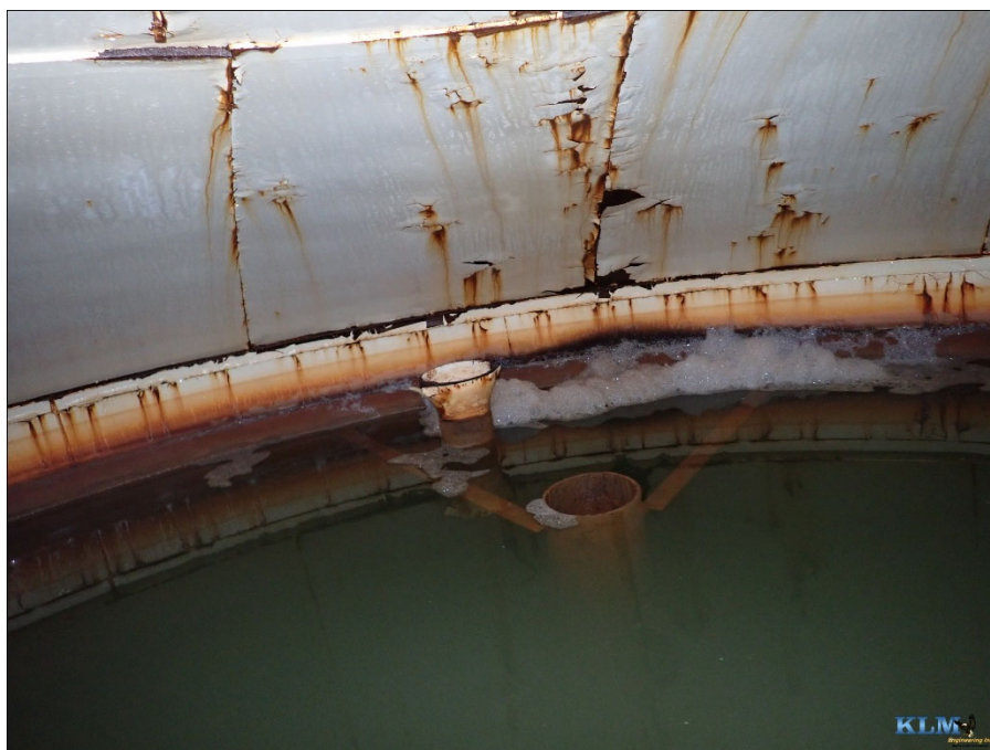
Photo No. 6 Overflow pipe and fill pipe
