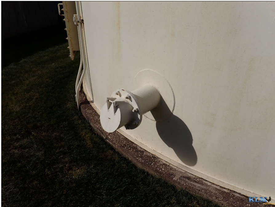
Photo No. 32 Overflow discharge
