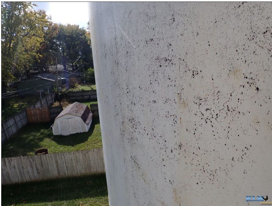
Photo No. 26 Shell coating condition
