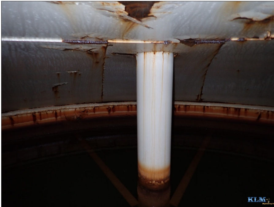
Photo No. 2 Roof condition and aeration pipe
