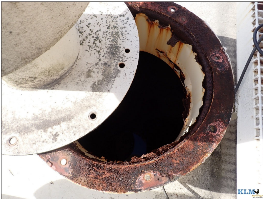
Photo No. 16 Corrosion on vent collar
