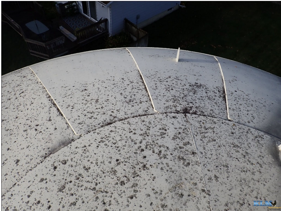
Photo No. 24 Roof coating condition
