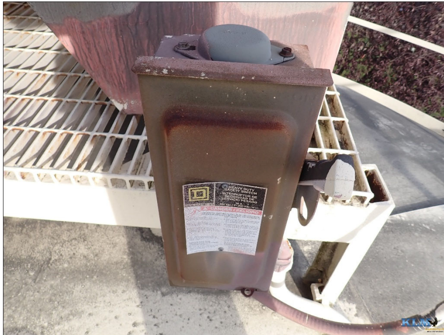
Photo No. 21 Electrical disconnect
