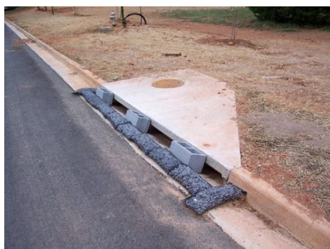
Typical rock bag inlet protection installation. Photo credit: Barry Tanning, Tetra Tech
