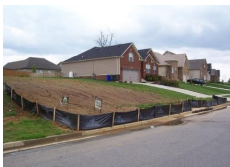
Site with properly installed silt fence. Note that fence posts are installed on the downhill side of the fabric. Photo credit: Barry Tanning, Tetra Tech
