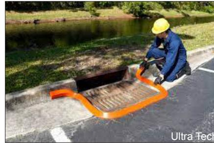
**Berms:** Manufactured berms can be used if grading is adequate and there are relatively smooth drainage surfaces. They can encircle a storm drain, allowing water to pond for later collection or diversion to the sanitary sewer.
