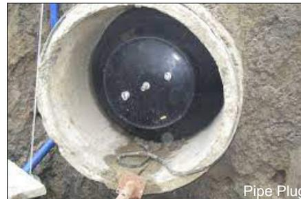
**Inflatable Pipe Plug:** The plugs are inserted into a storm drain pipe and inflated for a tight fit to prevent washwater from entering the pipe. Washwater is collected in the storm drain sump and then pumped to a holding tank or sanitary sewer.
