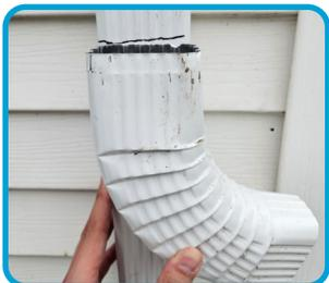
Cut the downspout with a reciprocating saw like a Sawzall or a hack saw. Make sure the cut is straight.
