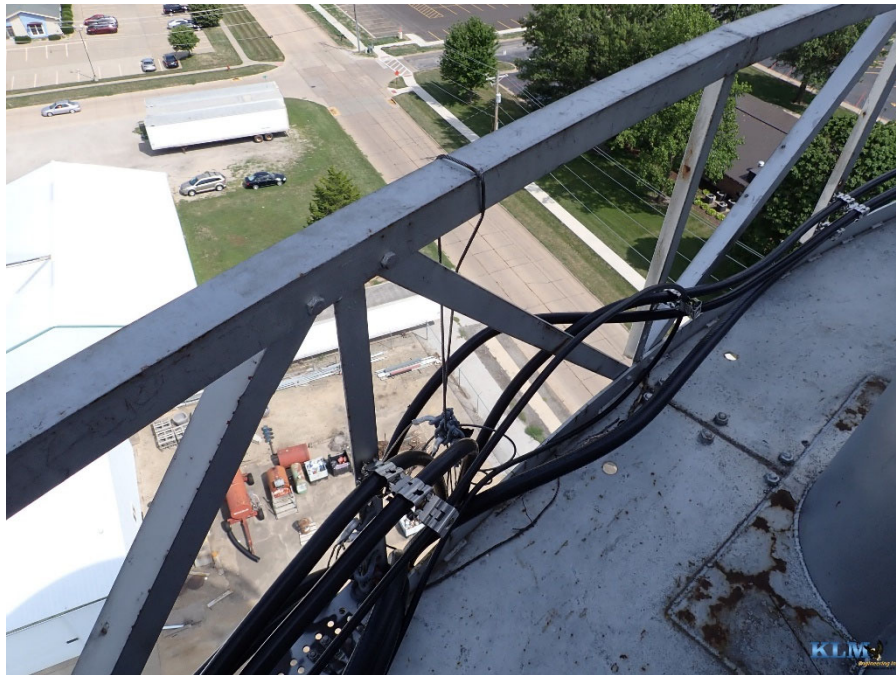
Photo No. 34 Balcony platform and handrail
