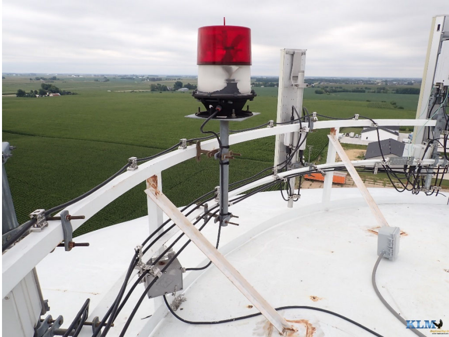
Photo No. 57 Roof and aviation light conditions
