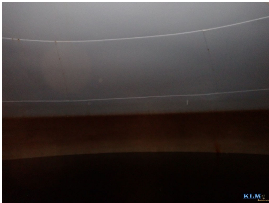
Photo No. 14 Roof coating conditions
