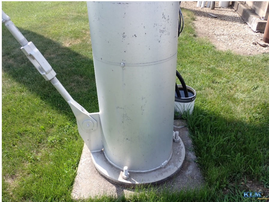
Photo No. 44 Typical conditions of column foundation
