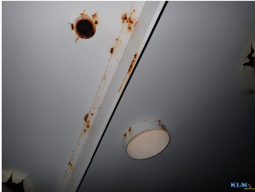
Photo No. 11 Interior roof conditions
