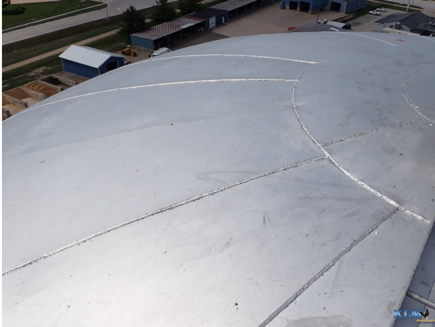
Photo No. 27 Roof coating conditions
