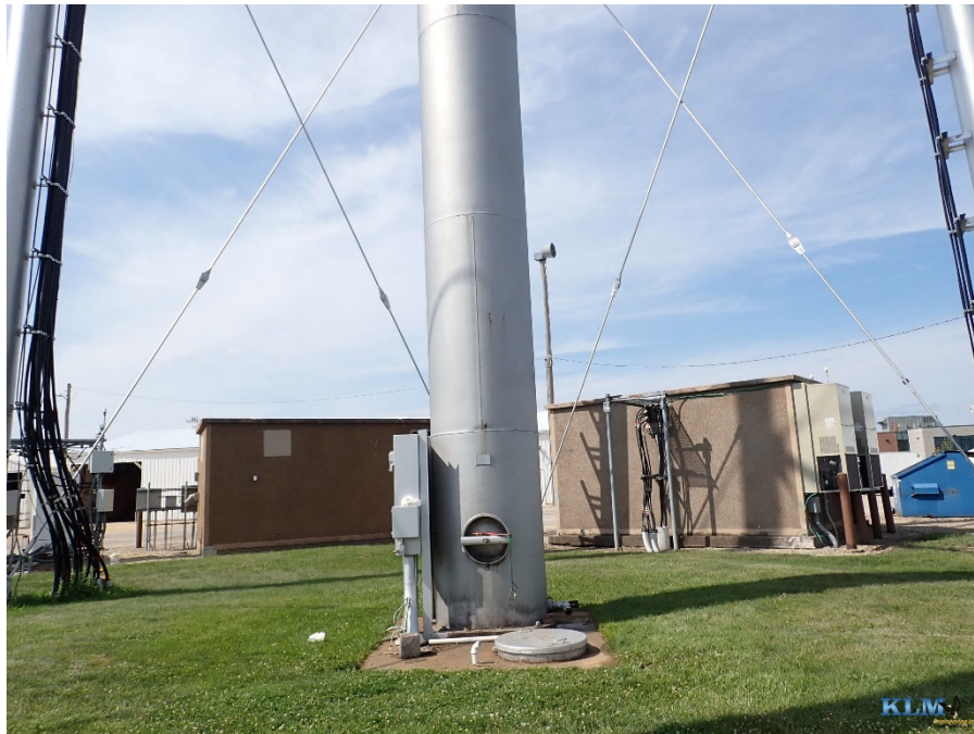
Photo No. 42 Wet riser conditions with manway visible
