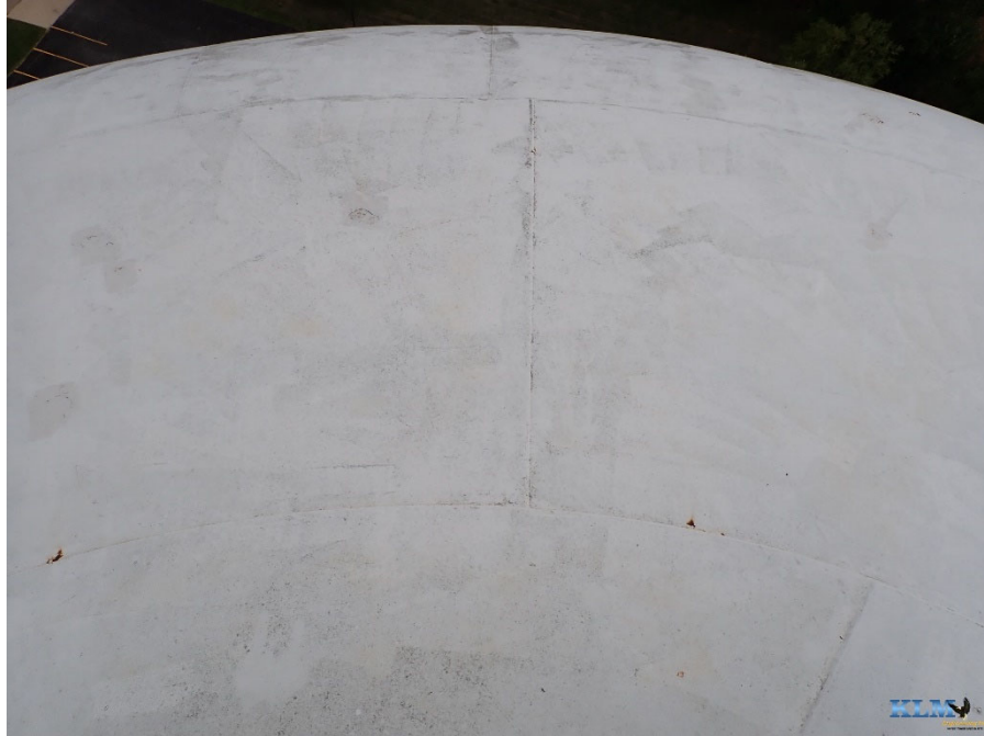
Photo No. 63 Exterior roof coating conditions
