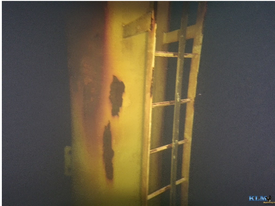
Photo No. 17 Drywell tube conditions below HWL
