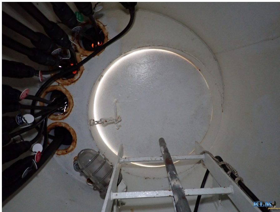
Photo No. 34 Top of drywell tube conditions
