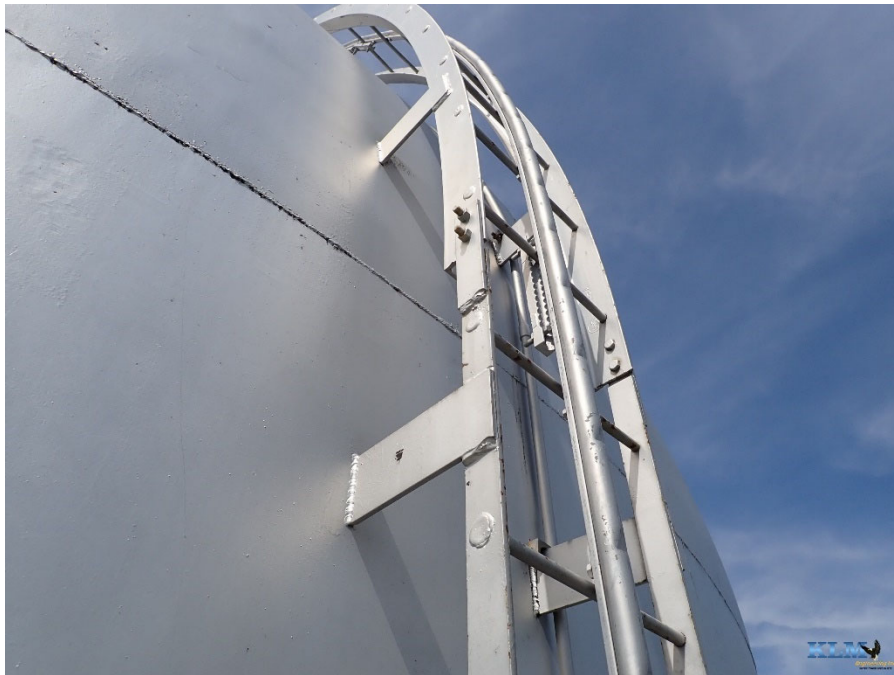
Photo No. 30 Roof access ladder
