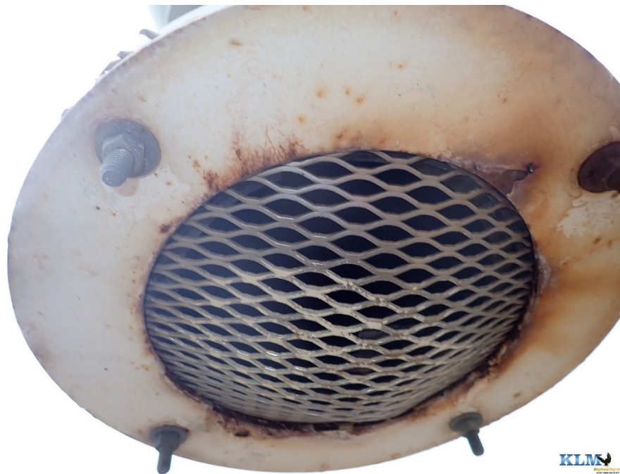
Photo No. 72 Overflow pipe screening conditions
