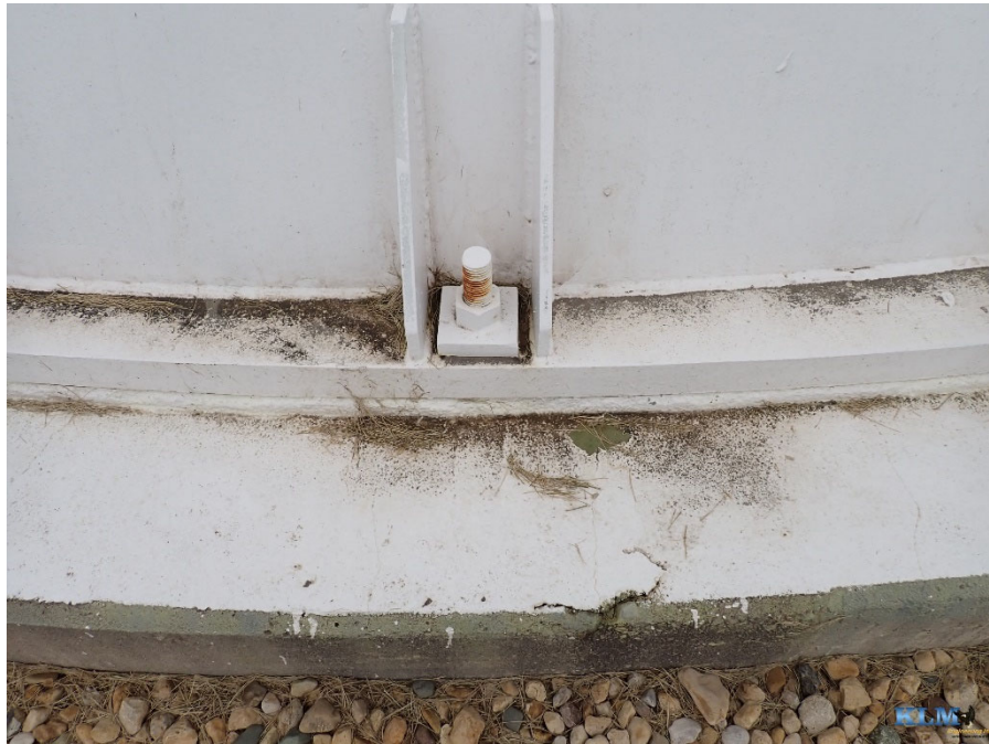
Photo No. 71 Typical conditions of ring foundation
