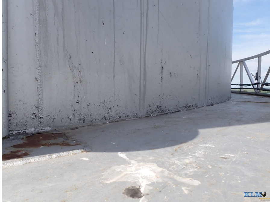
Photo No. 35 Balcony platform conditions
