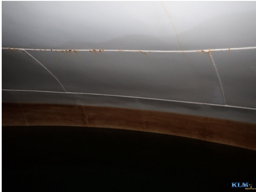
Photo No. 13 Roof conditions
