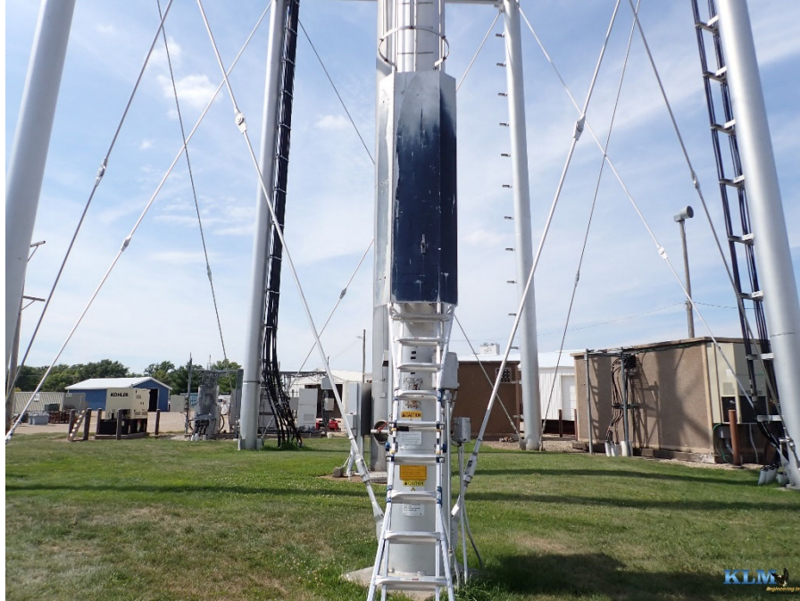
Photo No. 41 Column access ladder at grade
