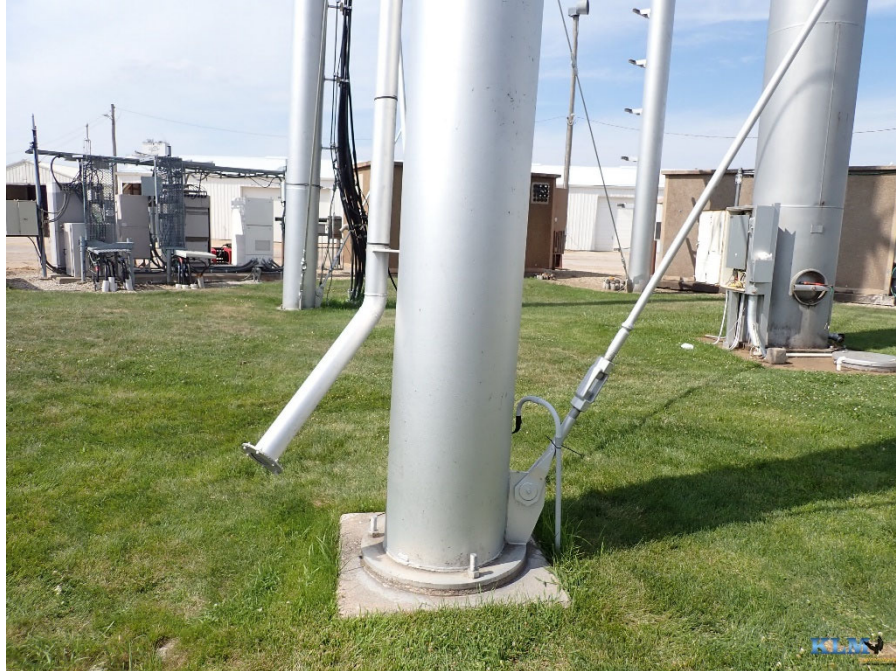
Photo No. 45 Column and overflow pipe outlet conditions
