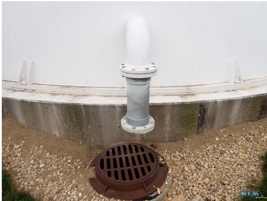
Photo No. 70 Overflow pipe outlet conditions
