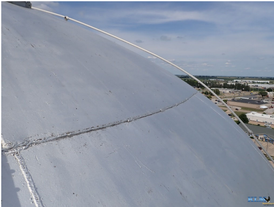
Photo No. 28 Roof coating conditions
