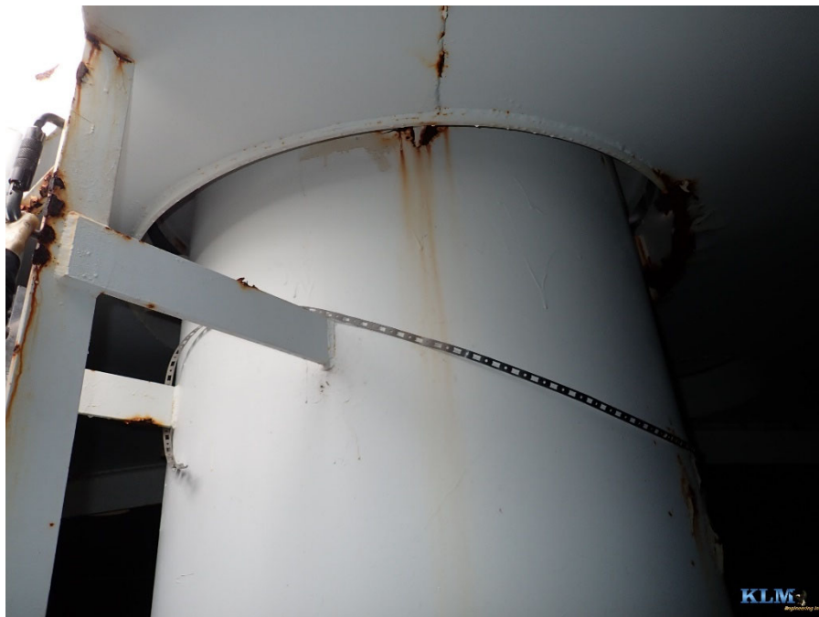
Photo No. 6 Roof conditions
