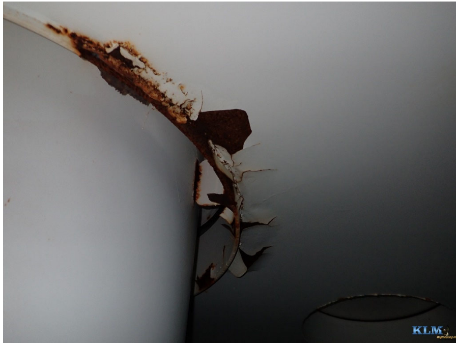
Photo No. 9 Top of drywell tube and roof conditions
