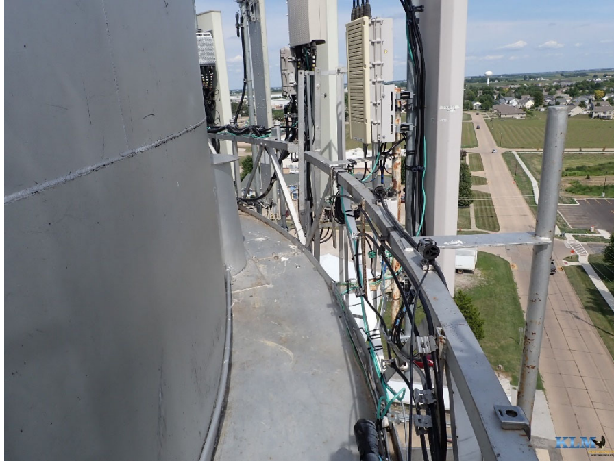
Photo No. 33 Balcony platform and handrail
