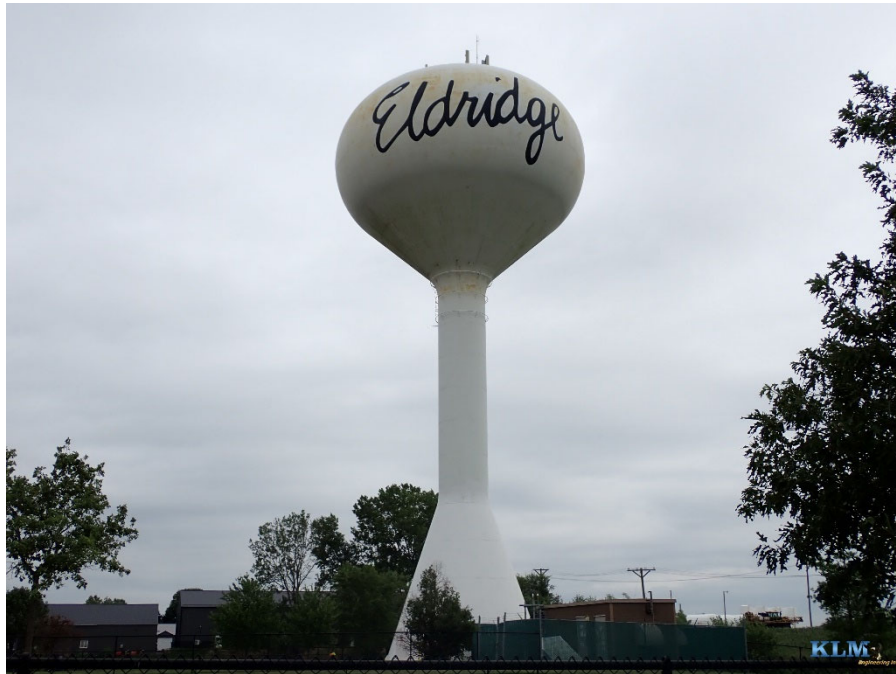
Photo No. 1 Overall view of the tower
