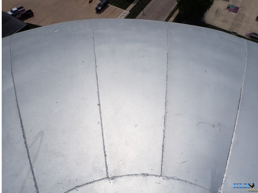
Photo No. 25 Roof coating conditions
