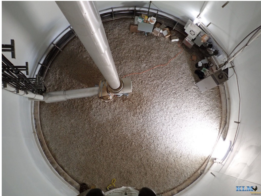
Photo No. 51 Overview of base cone area
