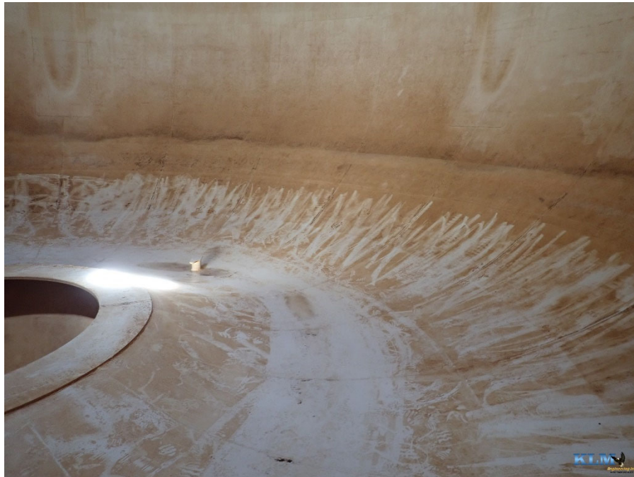
Photo No. 17 Bowl conditions after cleanout
