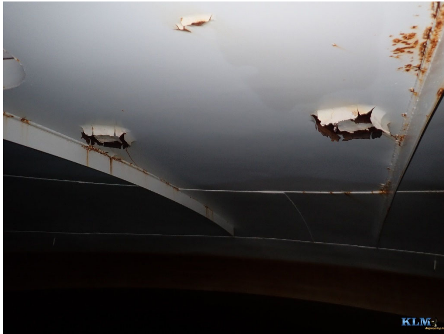
Photo No. 5 Interior roof conditions
