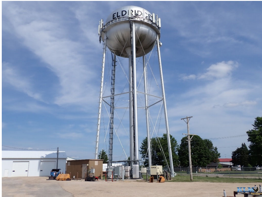
Photo No. 1 Overall view of tower
