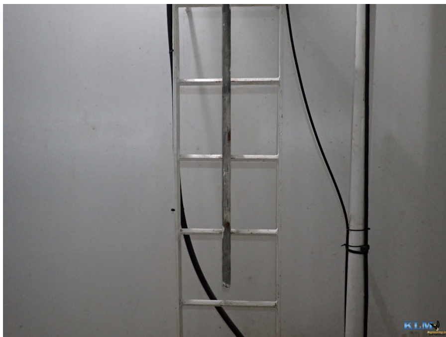
Photo No. 46 Typical pedestal conditions
