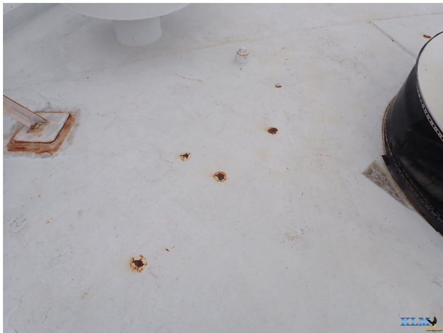
Photo No. 60 Roof conditions within handrail
