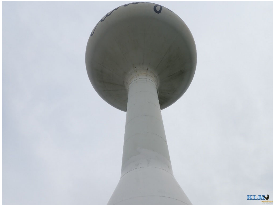
Photo No. 67 Overview of lower torus and pedestal
