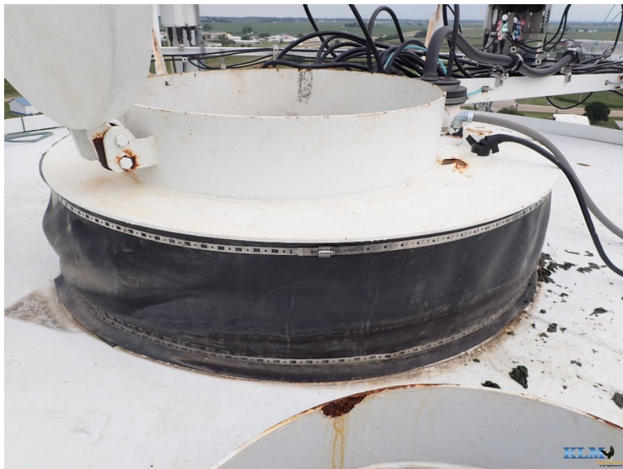
Photo No. 56 Dry access manway on roof
