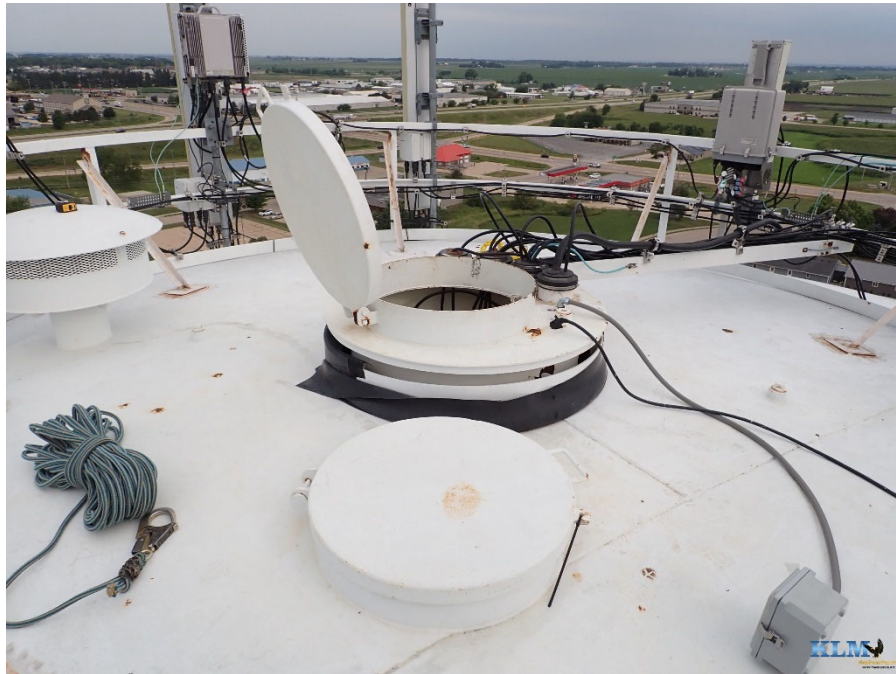
Photo No. 55 Roof exterior conditions
