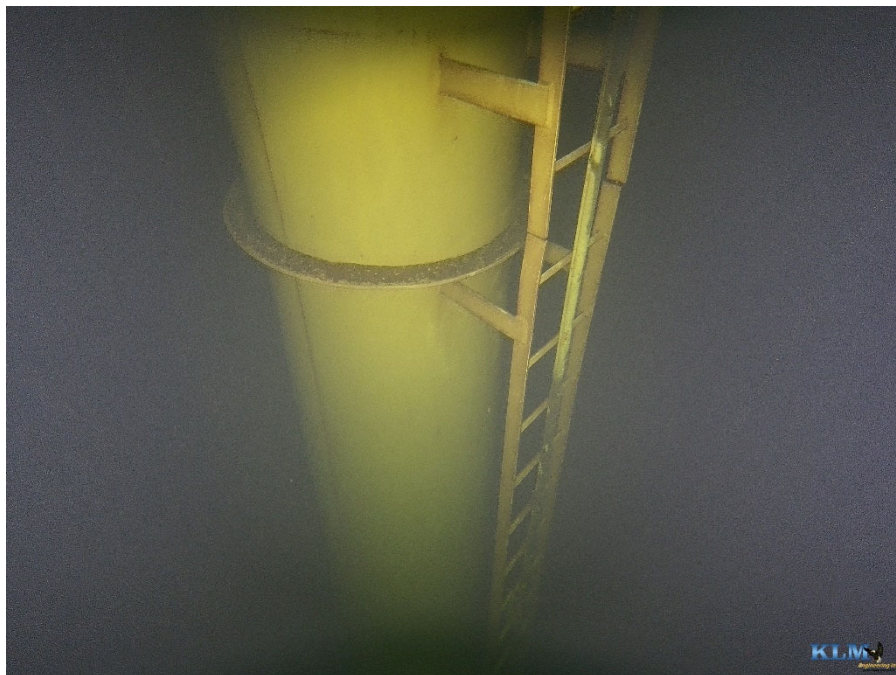
Photo No. 18 Drywell tube and ladder below HWL
