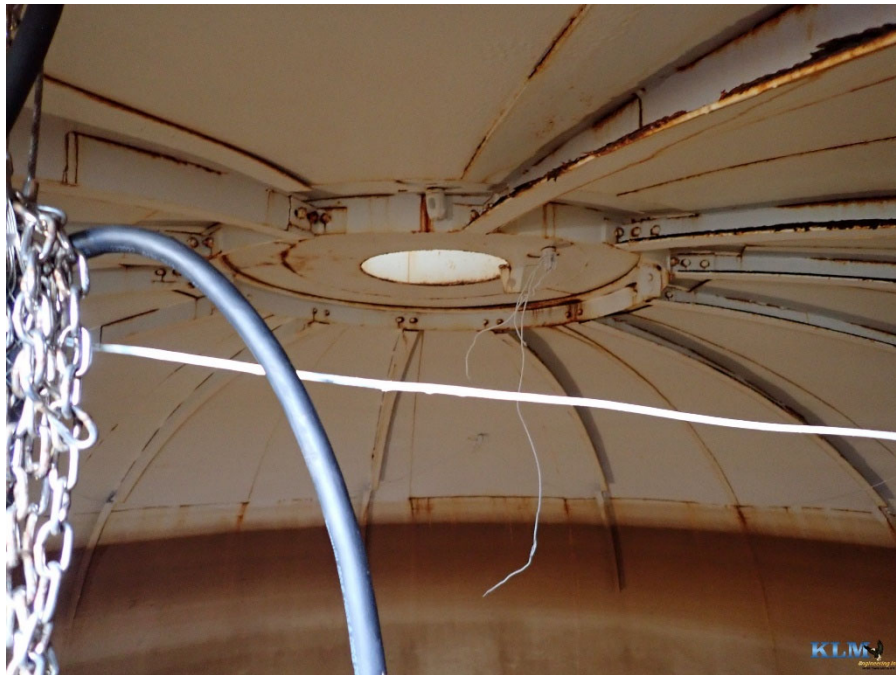
Photo No. 4 Rafters and compression ring
