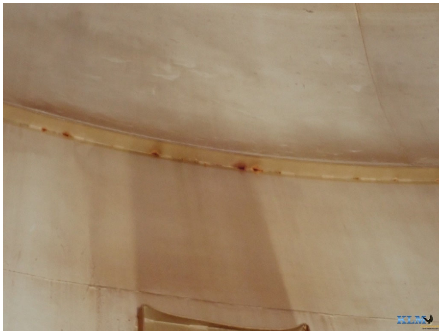
Photo No. 10 Shell stiffener ring
