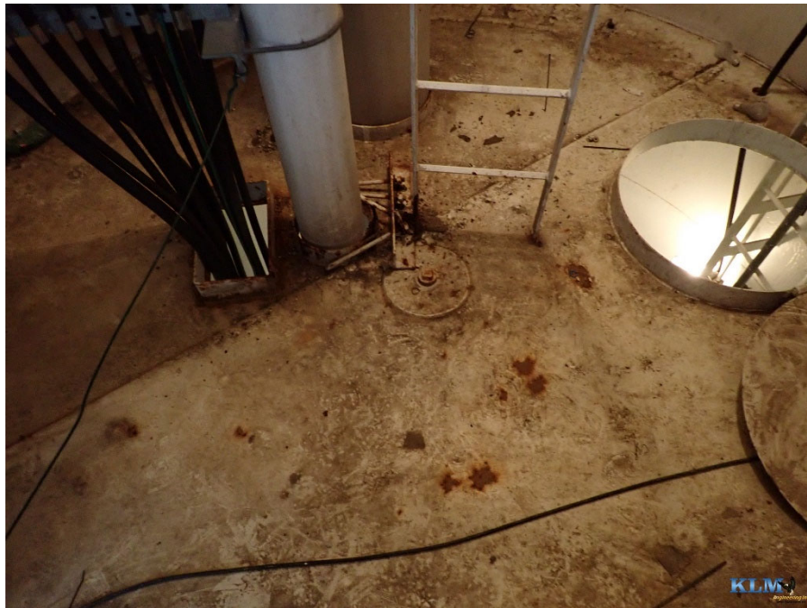
Photo No. 44 Top landing conditions
