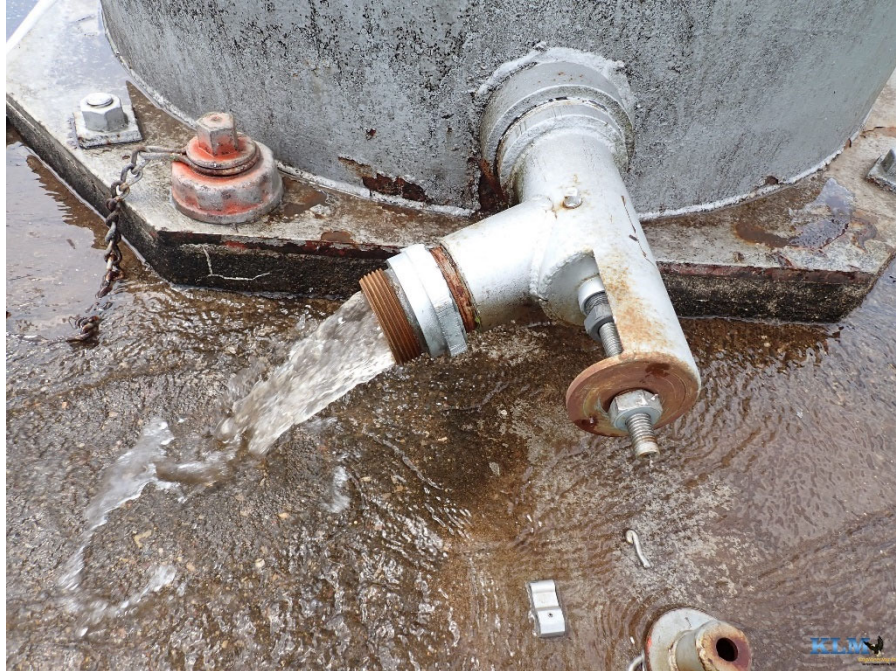
Photo No. 43 Wet riser foundation conditions with cleanout valve
