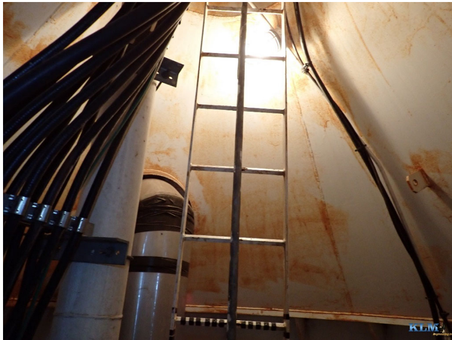
Photo No. 42 Bowl conditions with fill pipe and overflow pipe visible
