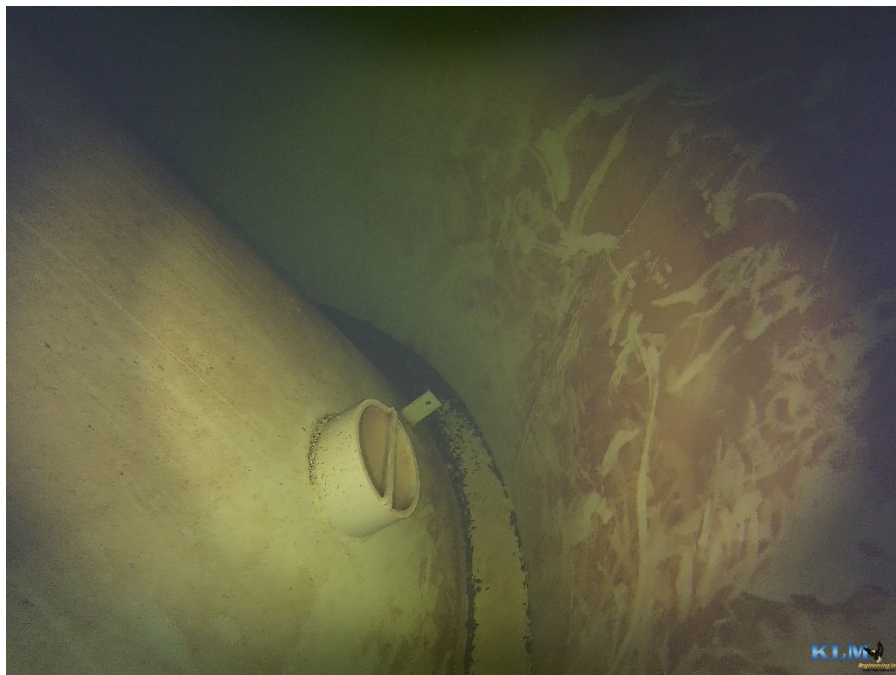
Photo No. 30 Bowl conditions with fill pipe visible
