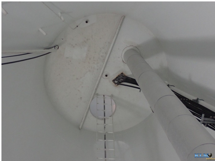
Photo No. 52 Base cone conditions looking up at bottom landing
