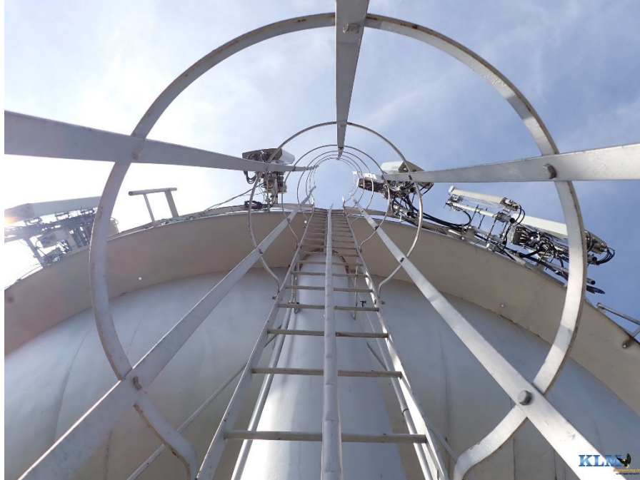
Photo No. 39 Column access ladder
