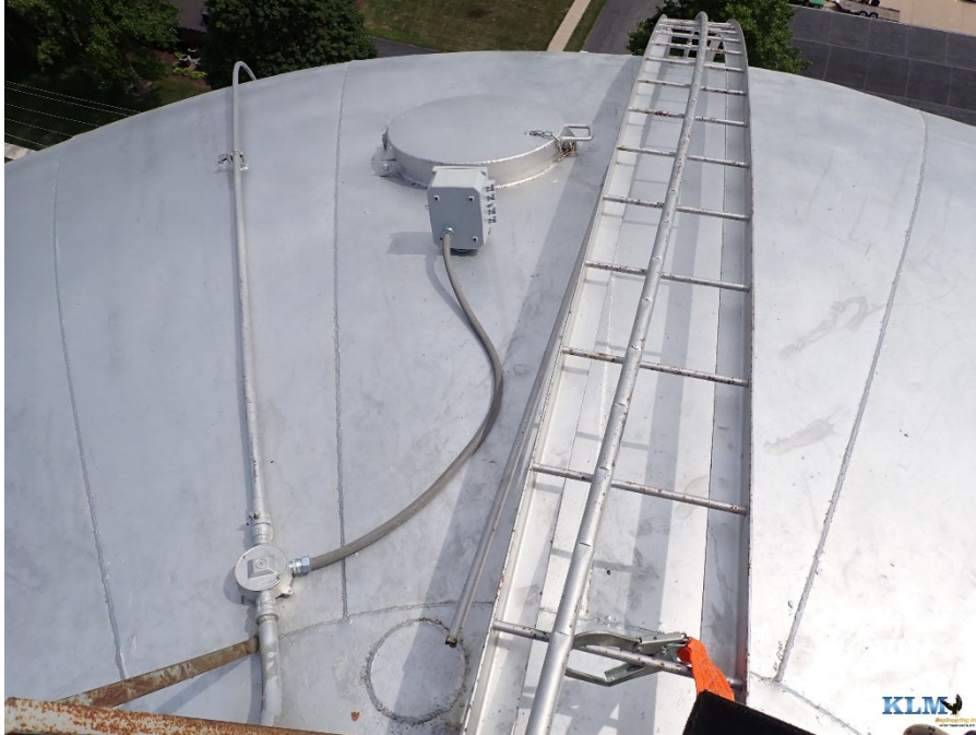
Photo No. 29 Roof coating conditions
