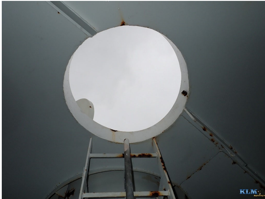
Photo No. 3 Roof and manway conditions
