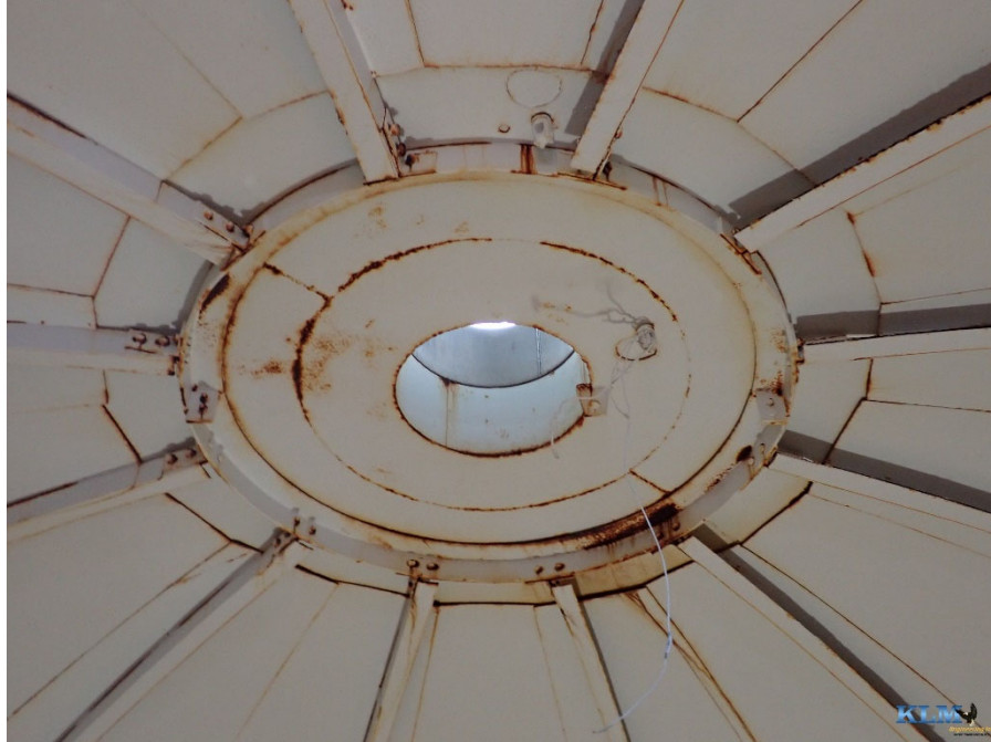
Photo No. 3 Interior roof conditions
