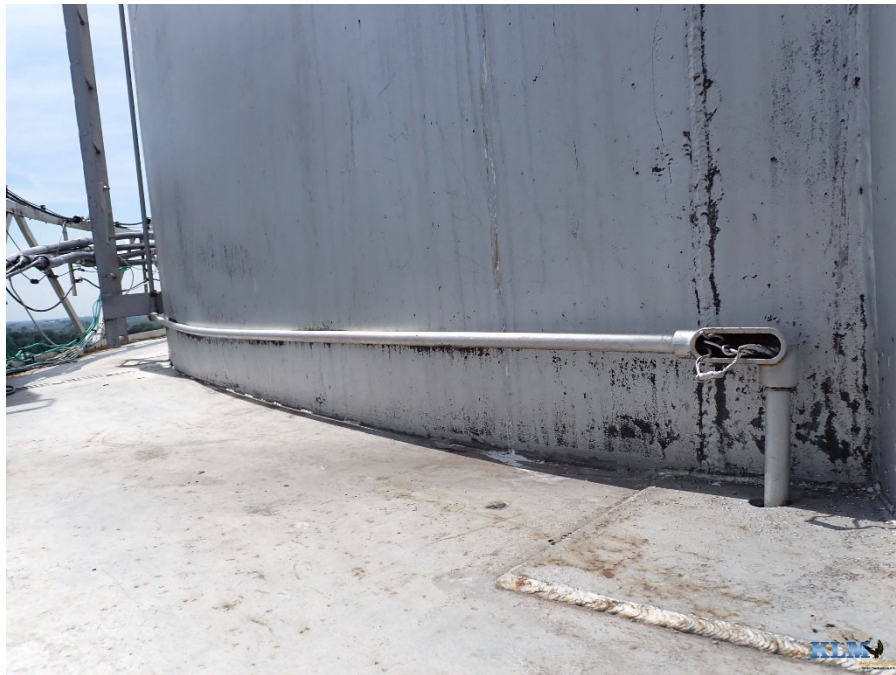
Photo No. 36 Balcony platform conditions
