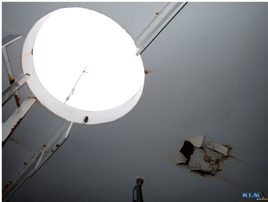
Photo No. 2 Interior roof conditions
