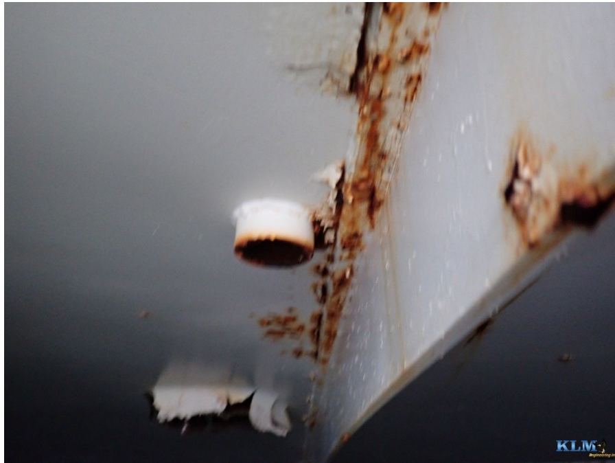
Photo No. 7 Roof with rafter and rigging coupling visible
