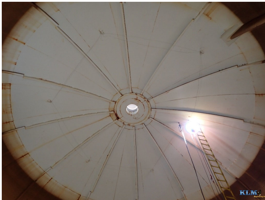
Photo No. 2 View of interior roof
