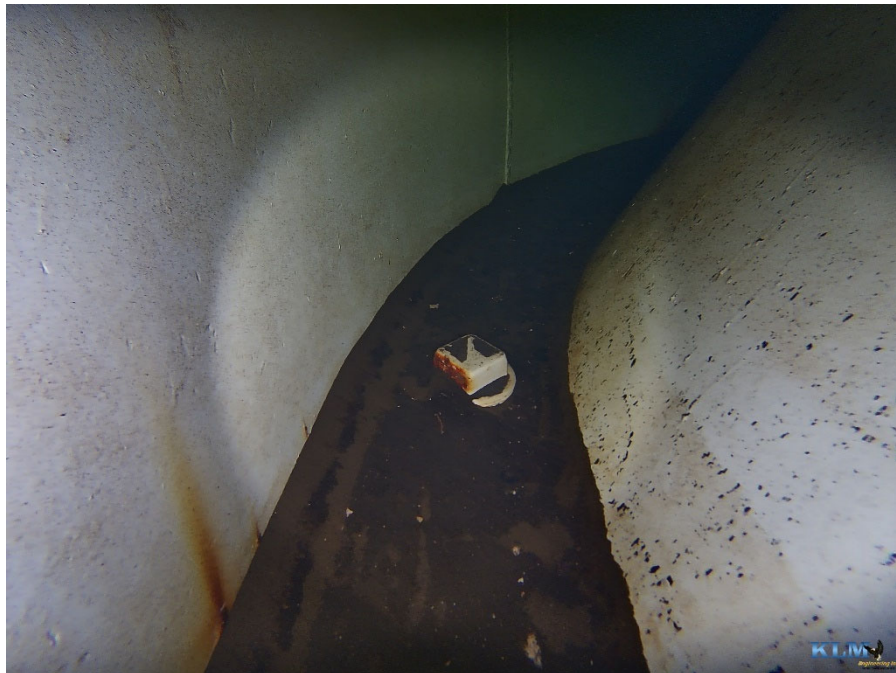
Photo No. 32 Bowl conditions with bowl drain plug and sediment visible
