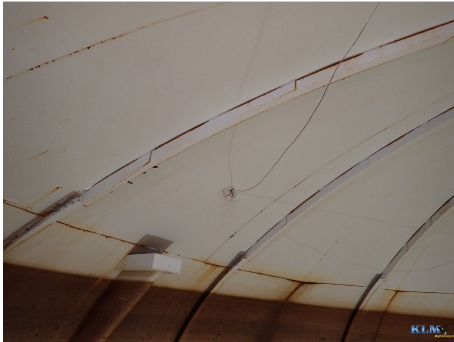
Photo No. 5 Roof and upper torus
