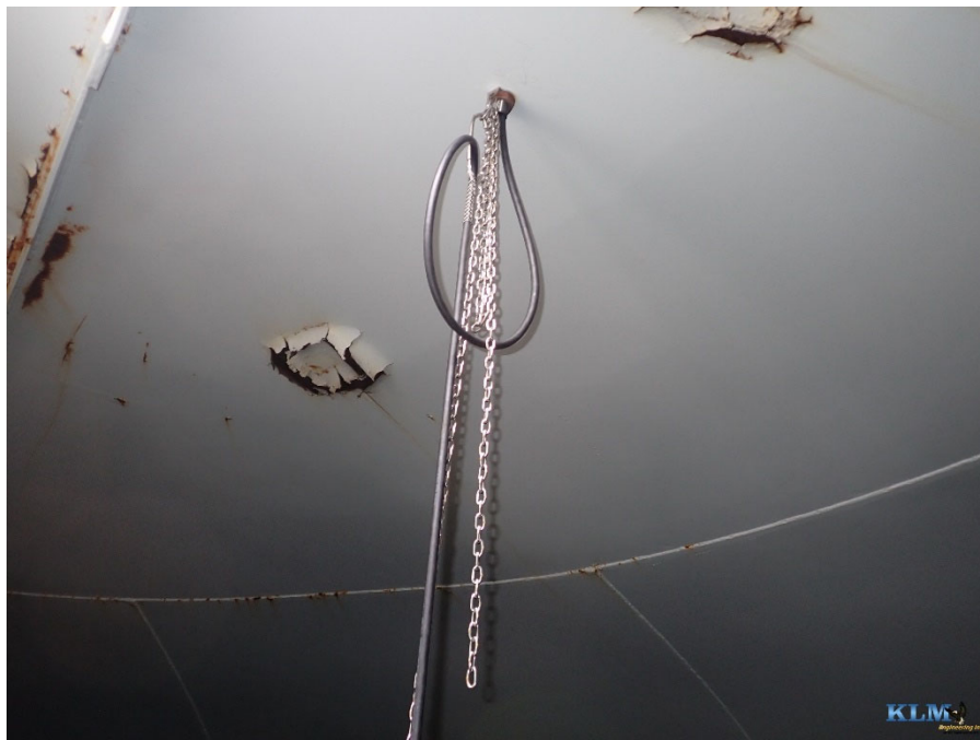
Photo No. 4 Coating conditions on roof
