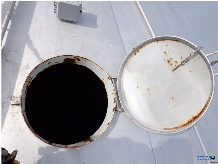
Photo No. 24 Wet access manway
