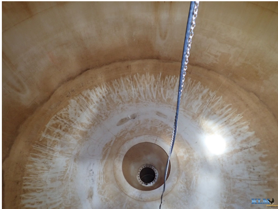
Photo No. 20 View of bowl after cleanout
