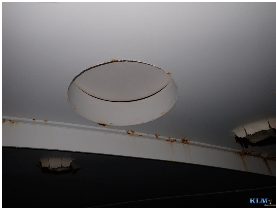
Photo No. 10 Roof conditions with vent and rafter visible
