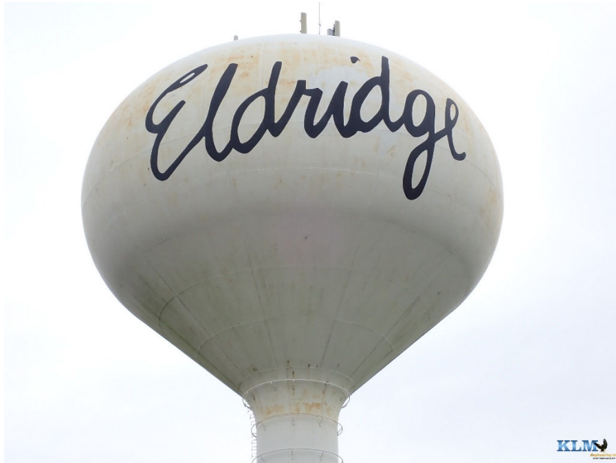
Photo No. 65 Water compartment conditions
