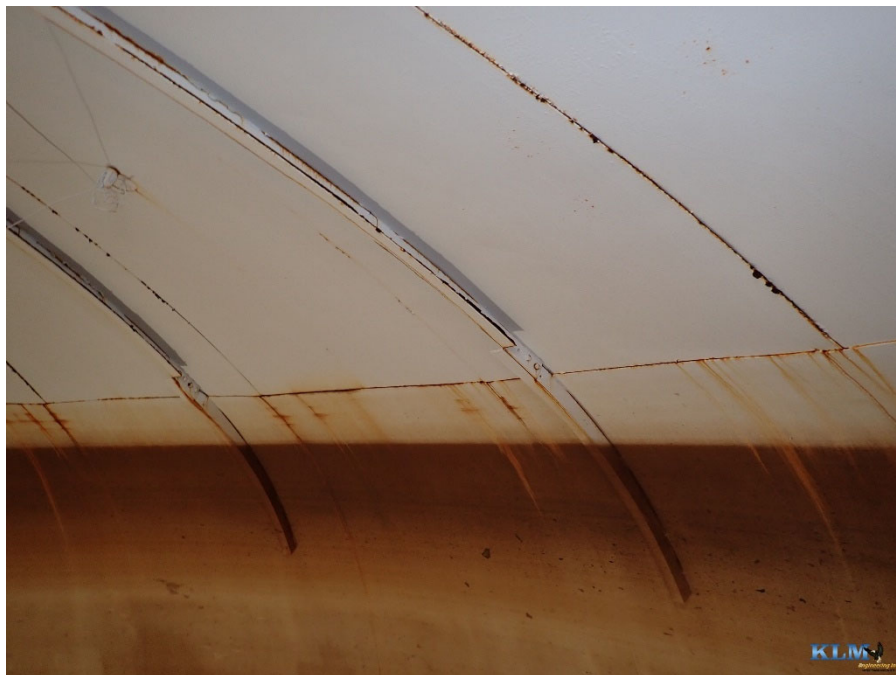
Photo No. 6 Roof and upper torus
