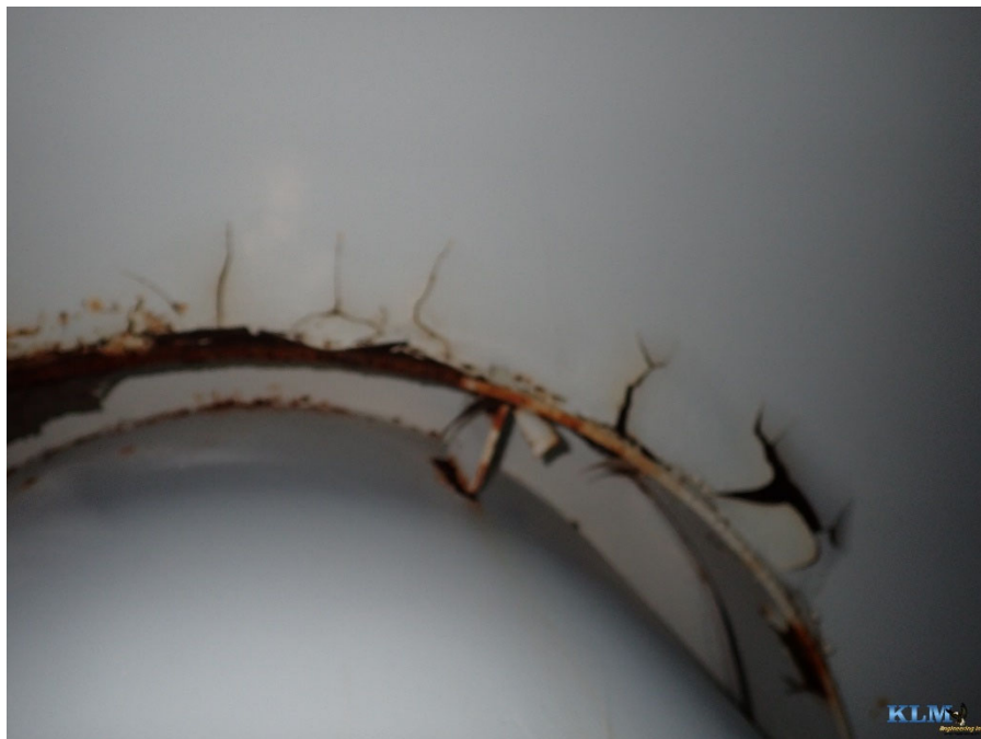
Photo No. 8 Interior roof at drywell tube connection
