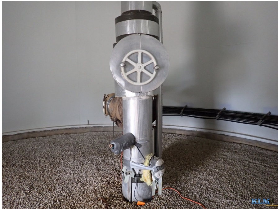
Photo No. 54 Base cone conditions
