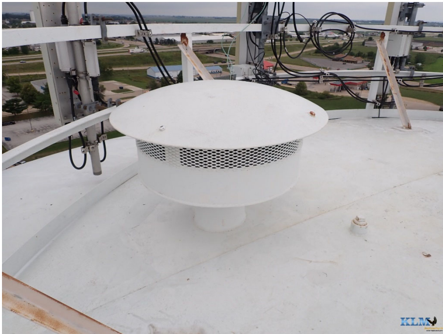
Photo No. 58 Roof and finial vent conditions
