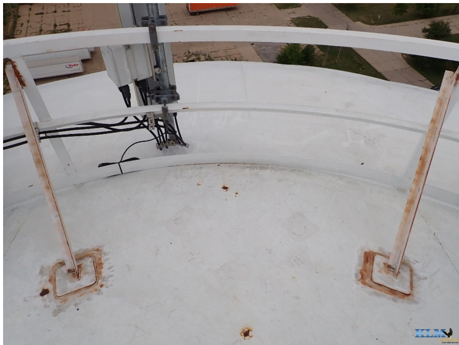
Photo No. 62 Handrail conditions on roof
