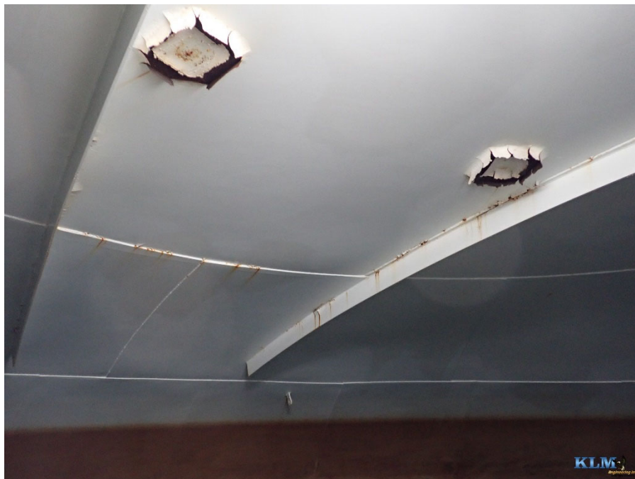
Photo No. 12 Coating conditions on roof
