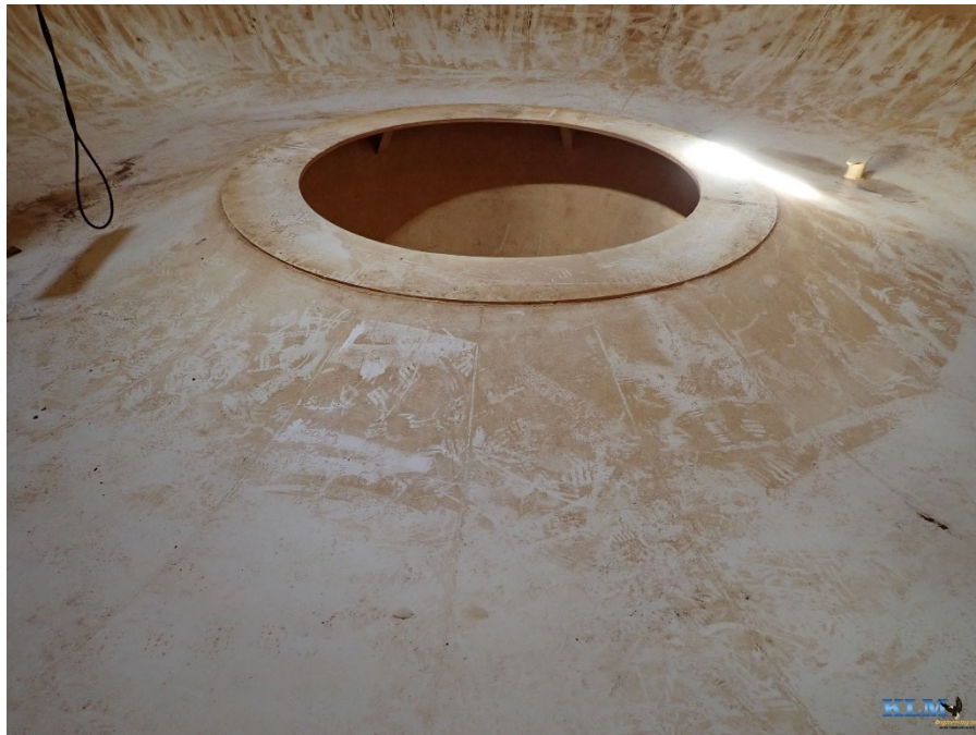
Photo No. 18 Bowl conditions after cleanout
