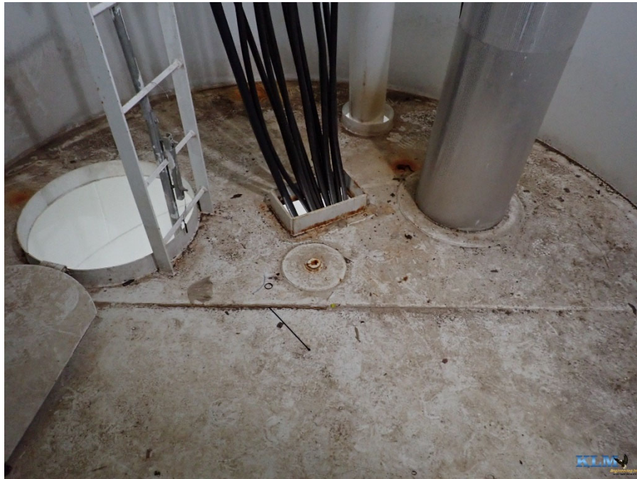
Photo No. 49 Bottom landing conditions
