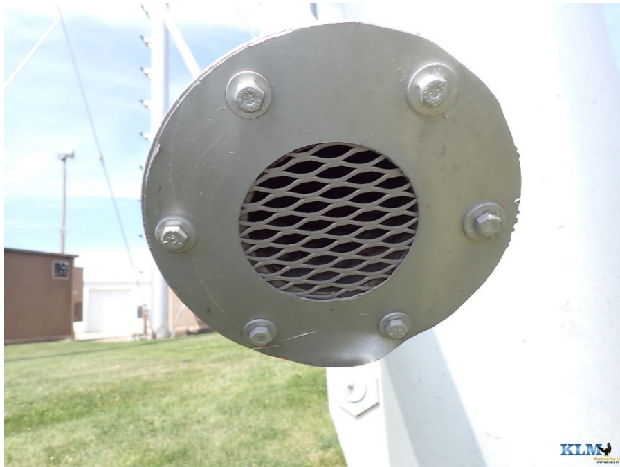
Photo No. 46 Overflow pipe screen conditions
