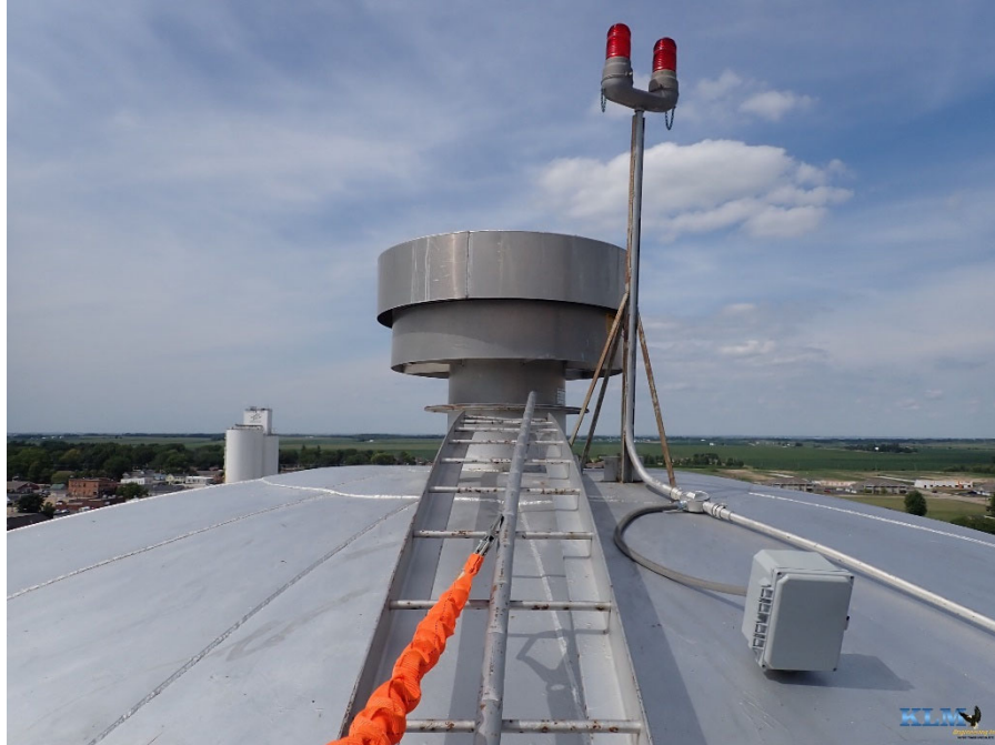
Photo No. 23 View of roof Finial vent and aviation light visible
